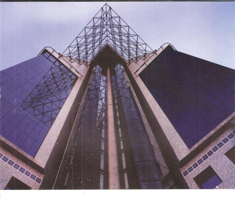
**7 & 8.** On either side of the atrium, five storeys of the building slopes backwards, creating an openness at the entry level. Framing the mass is an umbrella space frame.
